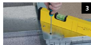
3 Level with the screws
